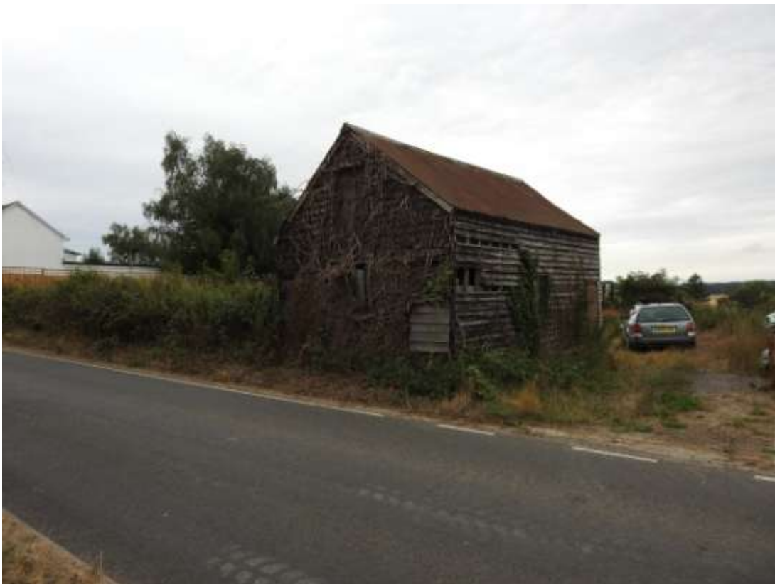
Plate 2. View of the site showing building to be demolished (looking south)
